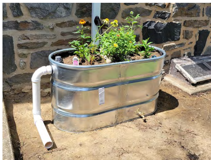
Downspout planter intercepts water previously directed to storm-water system
