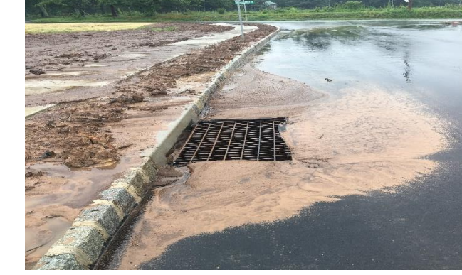
Virtually no inlet protection.
