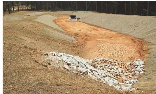
Large temporary sediment basin with skimmer, surrounding vegetation and mulching.
