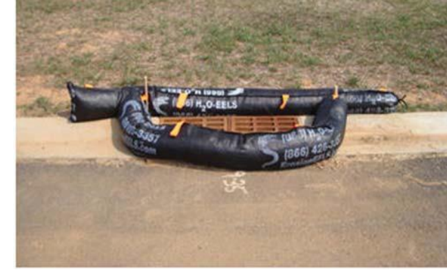
Excellent example of a well installed sediment barrier.
