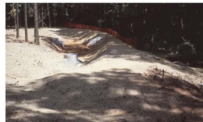
Well anchored mulch. Good coverage.
