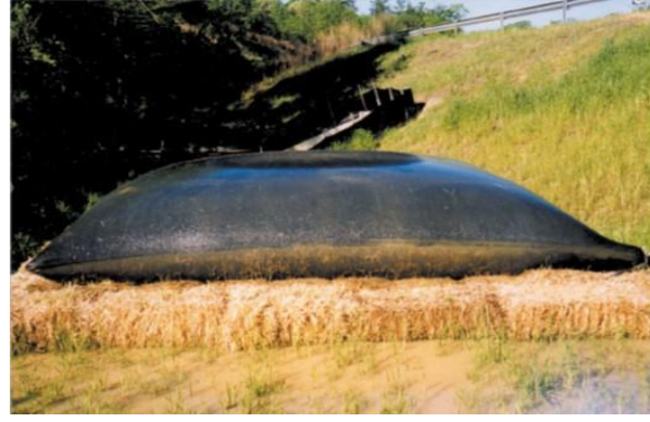
Sediment filter bag. Pumps water into the bag and filters out sediment. Situated atop hay bales to increase outflow efficiency. Photo: ACFEnvironmental.com
