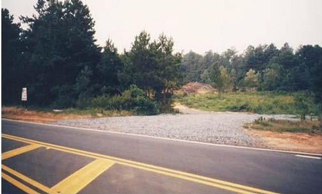
Excellent stone coverage. No mud tracking onto roadway.
