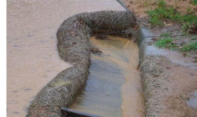
Improper maintenance has allowed properly installed straw wattle to be overwhelmed.
