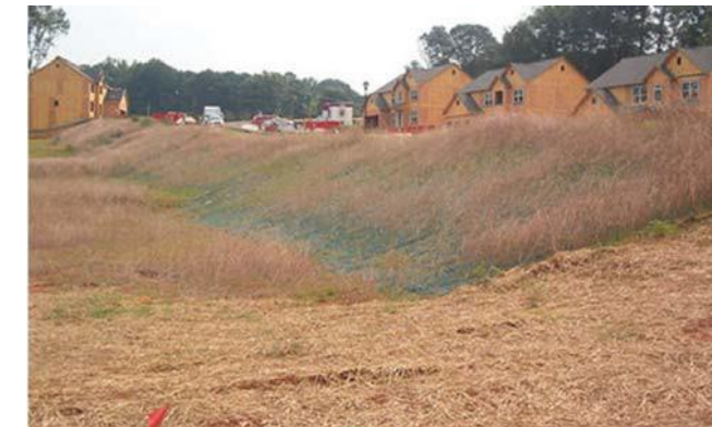
Some areas exposed. Temporary vegetative cover is dead.
