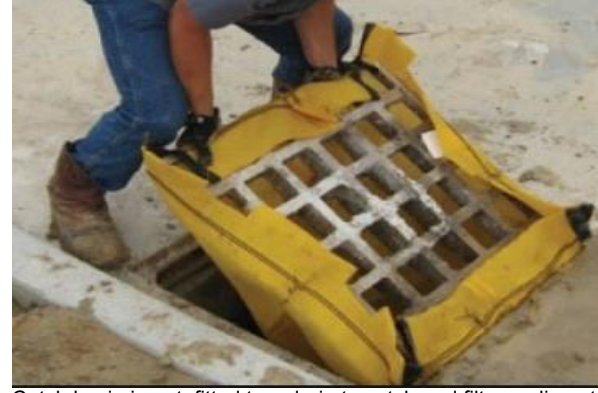
Catch basin insert, fitted to a drain to catch and filter sediment from construction site runoff. Watch for improper fitting around drain. Photo: concreteconstruction.net
