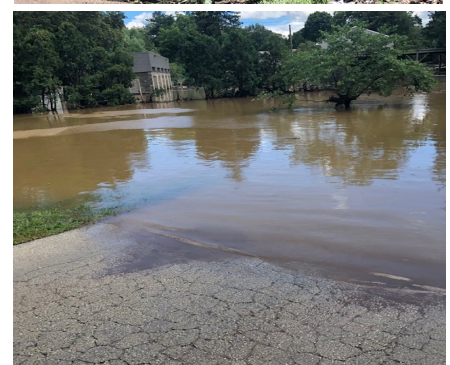
2009 Article by David Bjorkgren. Wreakage and flooding from Hurricane Isaias in 2020 in Merry Place Haverford Township. Photos above by Tim Denny
