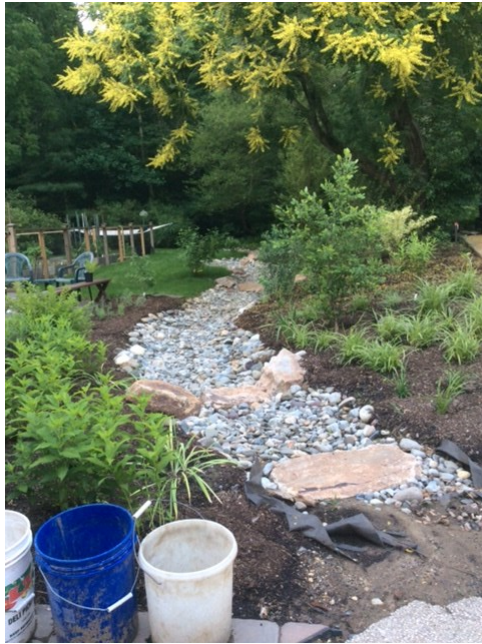
Some examples of the construction of private raingardens being constructed in Havertown. Top left: A attractive swale that drains water from the down spouts on the home to the garden. Top right: Rototilling to loosen soil to make it more hospitable for the growth of the young plants. Immediately to the right: Volunteers planting.
