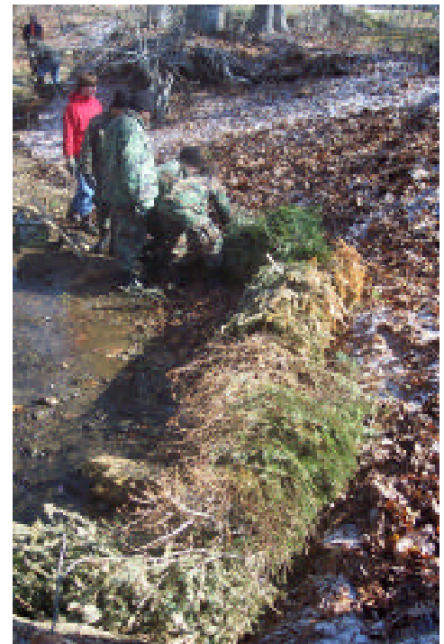
Cadets from Valley Forge Military Academy, scouts from Bryn Mawr Troop 19, and technical assistants from the Delaware Riverkeeper Network install Christmas trees as part of the community tree revegetation project at Clem Macrone Park in Garrett Hill.
