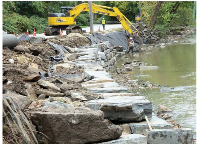
Stonewall construction along Scottdale Road
