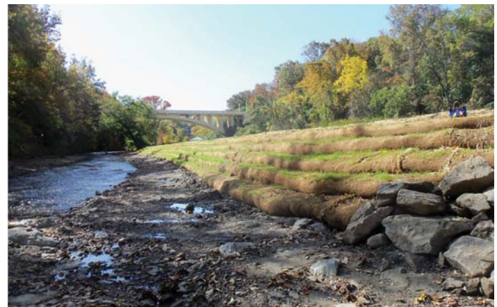
Vegetative Buffer at Kent Park Dam
