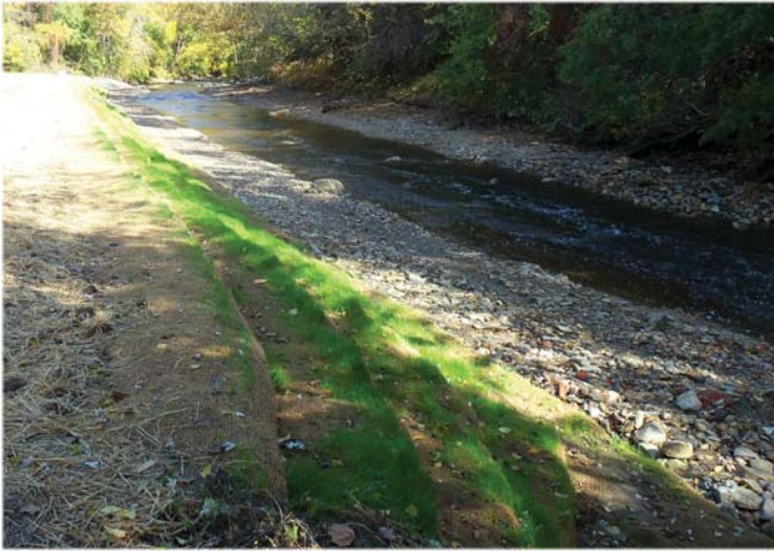
Looking downstream after Kent Park Dam has been removed
