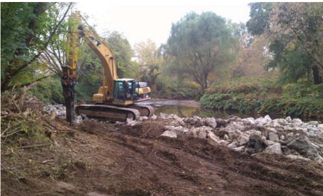
Reconstruction at the 12th Street dam site.
