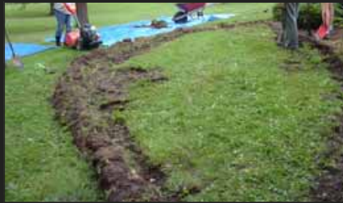
Build the berm with sod
