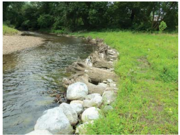
12th Street Dam, Darby: Root wads and rocks still stabilize the bank. The centrally located main channel meanders down stream. Grasses and tree stakes are growing on bank slope created by soil lifts.
