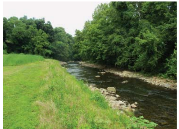
Kent Park (Looking downstream). The dam is still out!! Grasses and tree stakes are growing on bank slope created by soil lifts. Upper right: Tall grasses in the wetlands.
