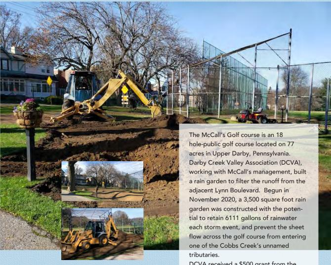
Research has shown that runoff from roadways, driveways can introduce pollutants into the waterways, and increase flooding downstream. Rain gardens are gardens constructed to capture stormwater. They are planted with water tolerant native plants. Rain gardens retain and filter stormwater runoff from impervious surfaces, such as driveways, parking lots and roadways, through plants and soils. This process reduces stormwater flow into creeks, removes pollutants and improves water quality.
